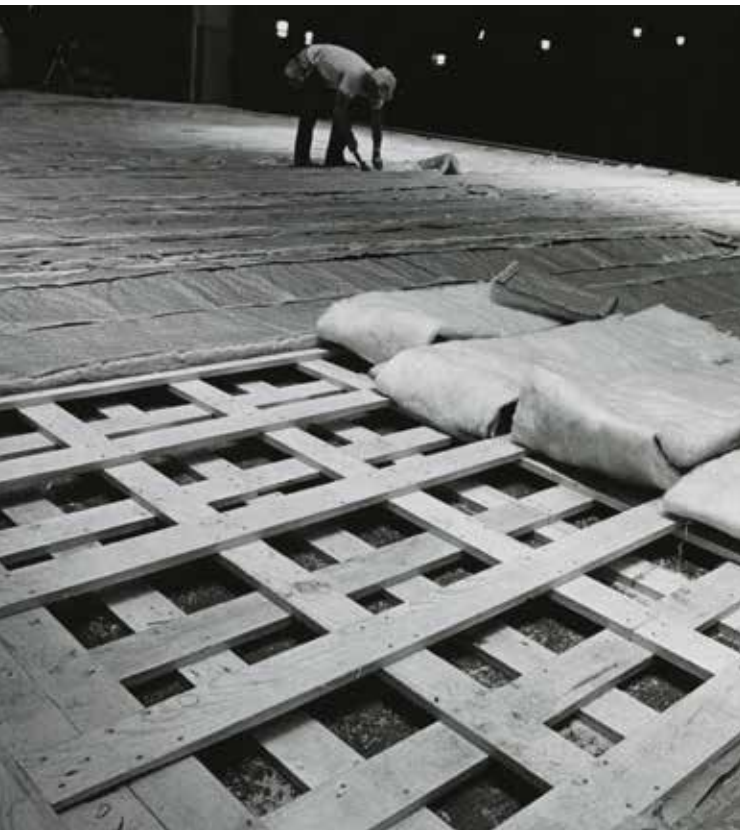
1975 installation of the “Balanchine basket weave” sprung-wood floor, duplicating what George Balanchine developed for the New York City Ballet.
