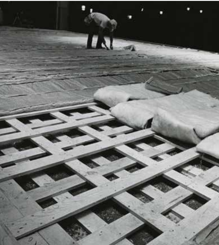
1975 installation of the “Balanchine basket weave” sprung-wood floor, duplicating what George Balanchine developed for the New York City Ballet.
